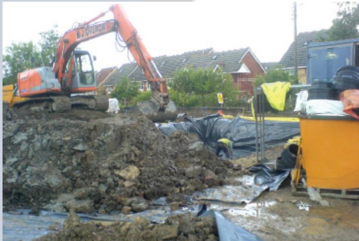
The soils were then back-filled into the pit as the groundworkers applied SpillAway Liquid Remediate and Dry Remediate directly to the soil.
